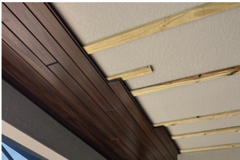
Installation of Synergy Wood with furring strips over drywall.
